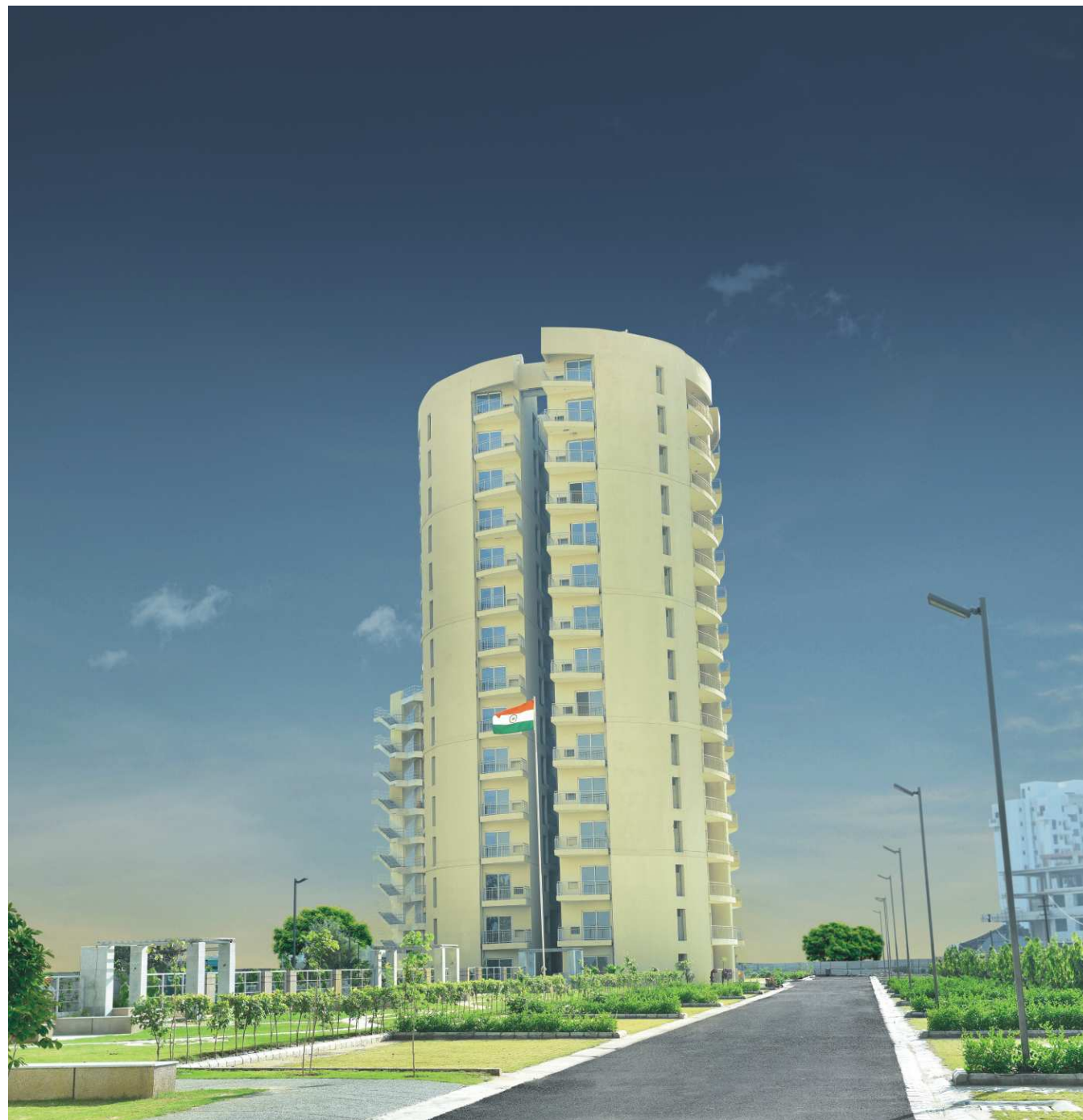
Actual image of ILD Greens Tower, Sector 37C, Gurgaon
